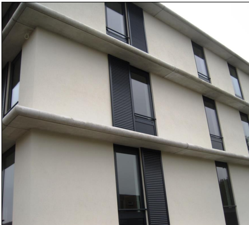
Appartementencomplex te Brunssum
